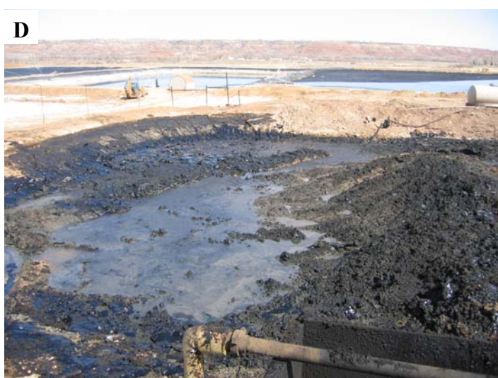
Figure 8. Commercial water disposal facility, used by Altamont-Bluebell-Cedar Rim field operators, near the town of Roosevelt. (A) Brine evaporation ponds. (B) Cement flats where oily sludge is skimmed off the top and sent to a centrifuge (C) where brine, solids, and oil are separated. (D) Reclamation of an evaporation pond.
