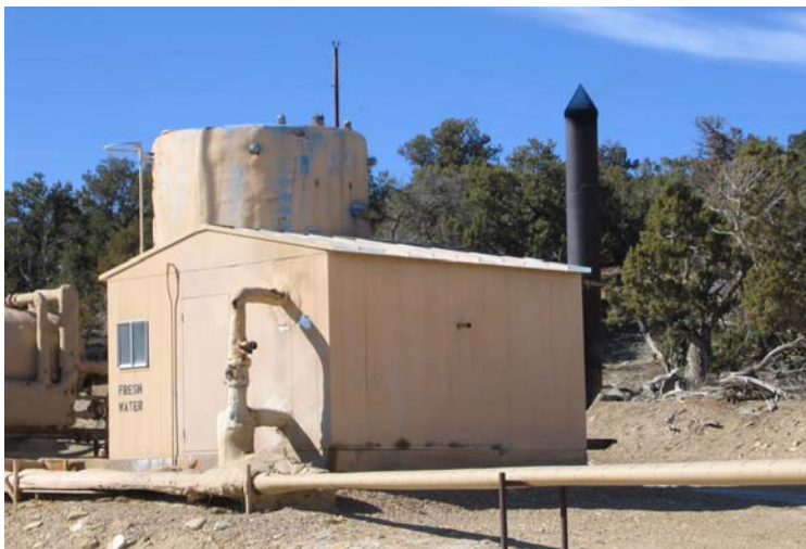
Figure 9. Heat treater with bird screen on the exhaust stack at the El Paso Production Oil and Gas Company Ute Fee 2-33C6, SW1/4SW1/4 section 33, T. 3 S., R. 6 W., UBLM, in Cedar Rim field.
