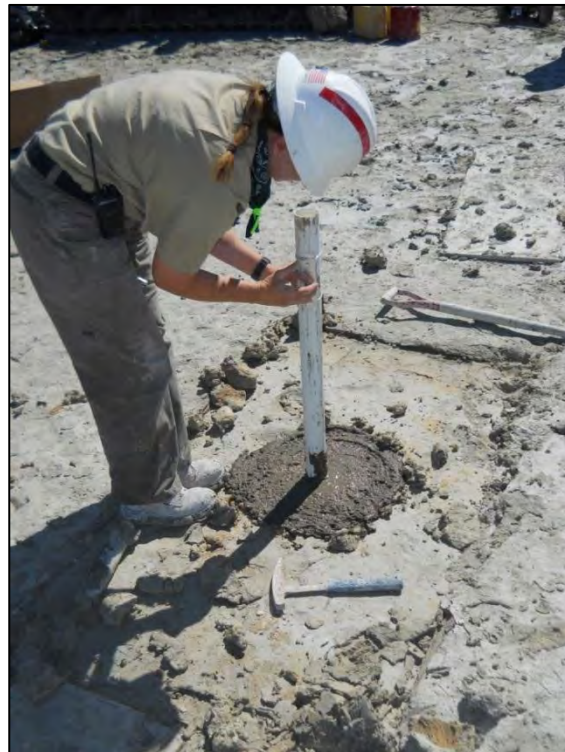
FIGURE 10.3 DIRECT PUSH HOLE CASED COMPLETION
