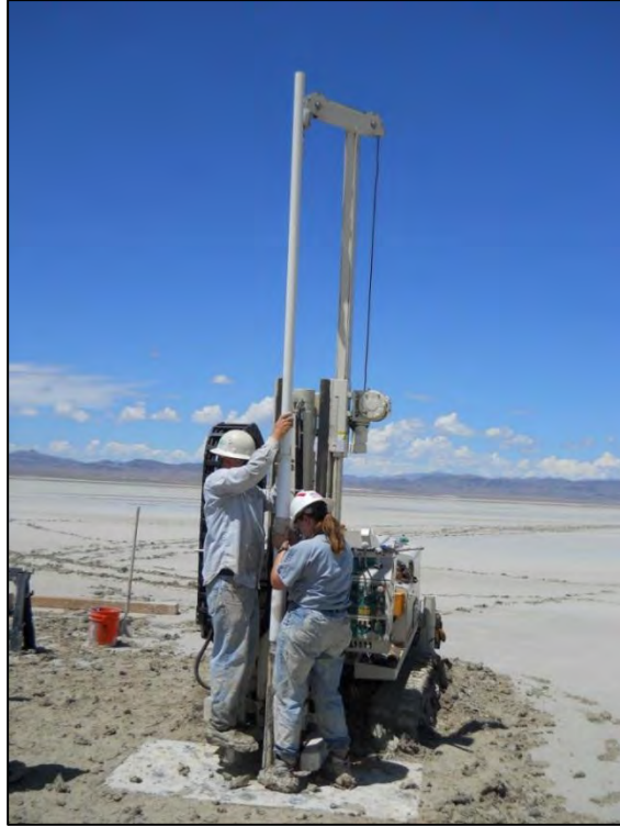
FIGURE 10. 2 PHOTO OF DIRECT PUSH HOLE CASING INSTALLATION
