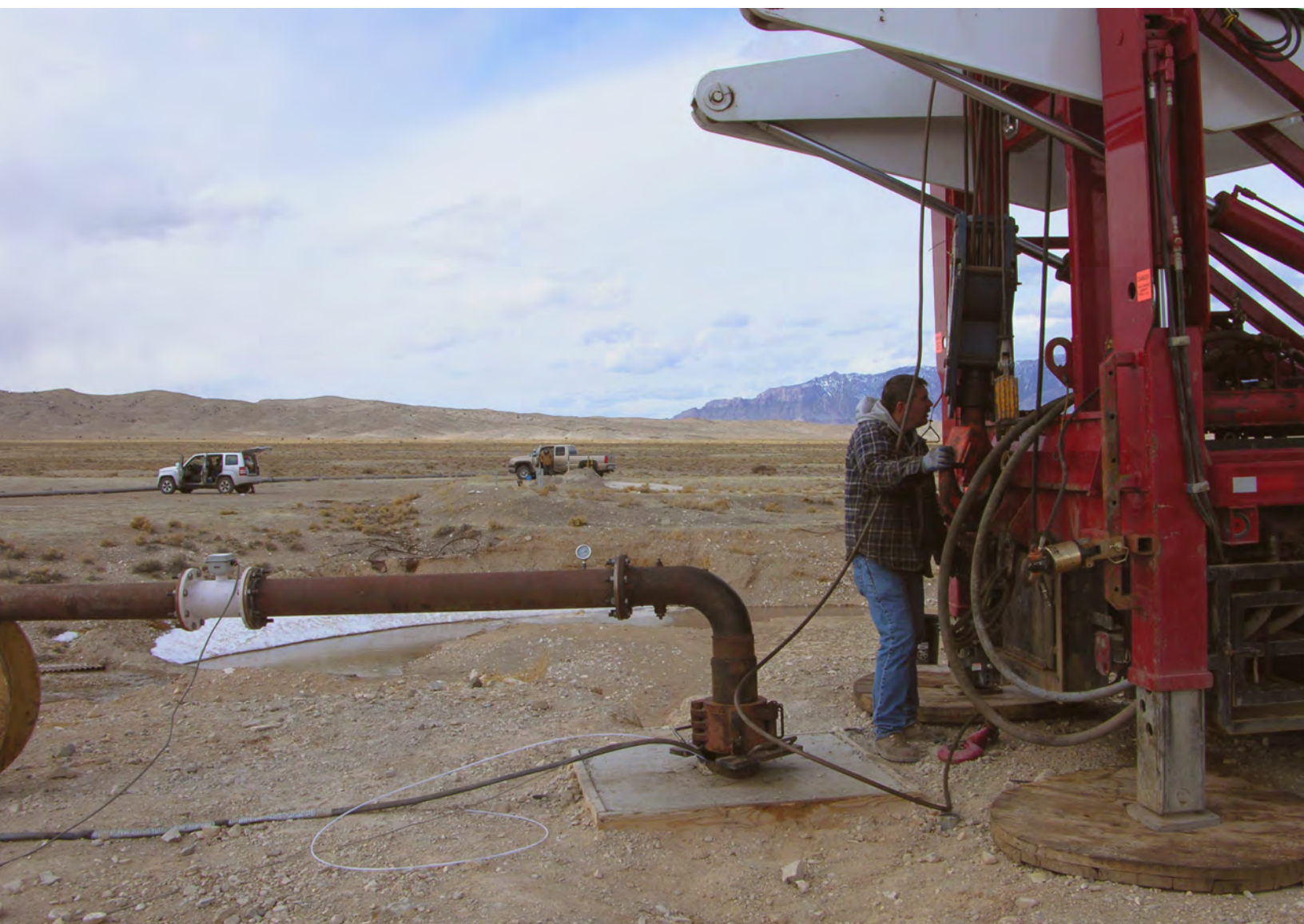
A contractor operates the pump rig at site 11 while UGS personnel measure water levels in observation wells in the background, March 2009.
