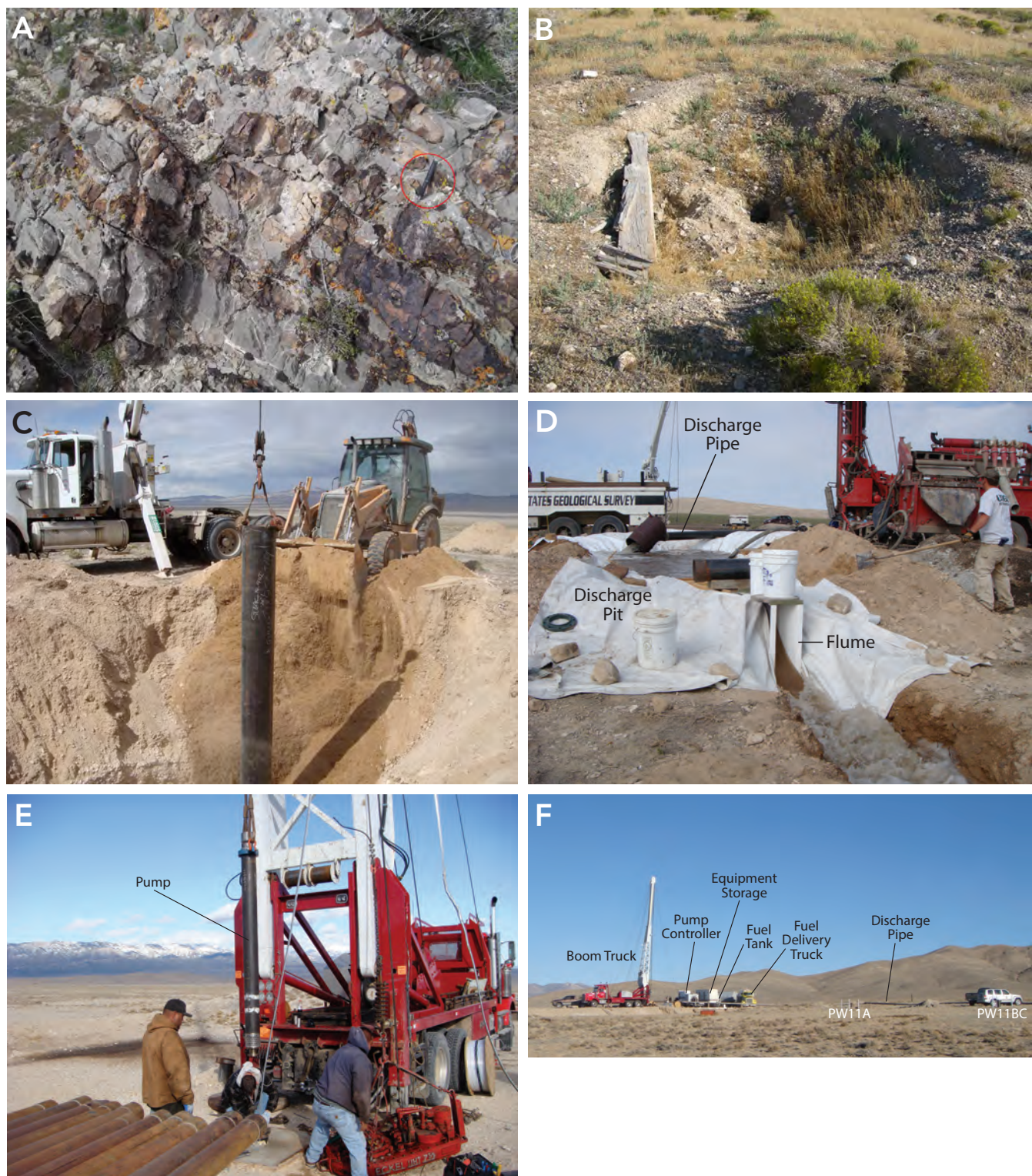
Figure 7.3. UGS aquifer-test site 11. A. The Permian-Mississippian Ely Limestone on north-south striking ridge northeast of site 11. The pumping and observation wells at this site are screened in this unit. Pencil (circled) is 5.5 inches (14 cm) long. B. View of well NPA-1B at site 11 before reconditioning. C. Installing new surface casing on well NPA-1B. D. Discharge pit and flume during the preliminary air-lift test of NPA-1B. E. Installing the pump into NPA-1B prior to the aquifer test. F. Equipment and monitoring sites during site 11 aquifer test.
